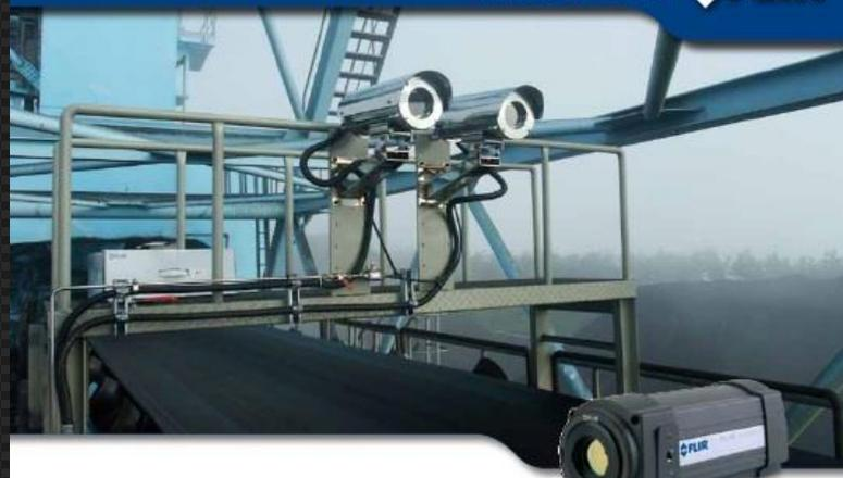
Thermal imaging cameras prevent fires at Korean coal power plant
