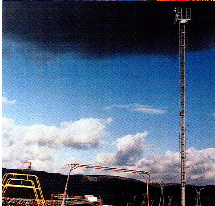
Continuous combustion detection to prevent spontaneous fires with a surveying ThermoVision™ by FLIR Systems
