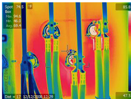
Thermal imaging cameras can be used to scan the entire system surrounding the wind turbines as well. One of these three phase connectors, the rightmost one, is much warmer than the rest. This defect was spotted and was repaired before a failure occurred.
