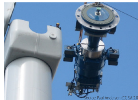
This huge 12 ton gearbox and disk brake assembly is lifted with a crane to a height of 60 meters to be mounted in this wind turbine nacelle.
